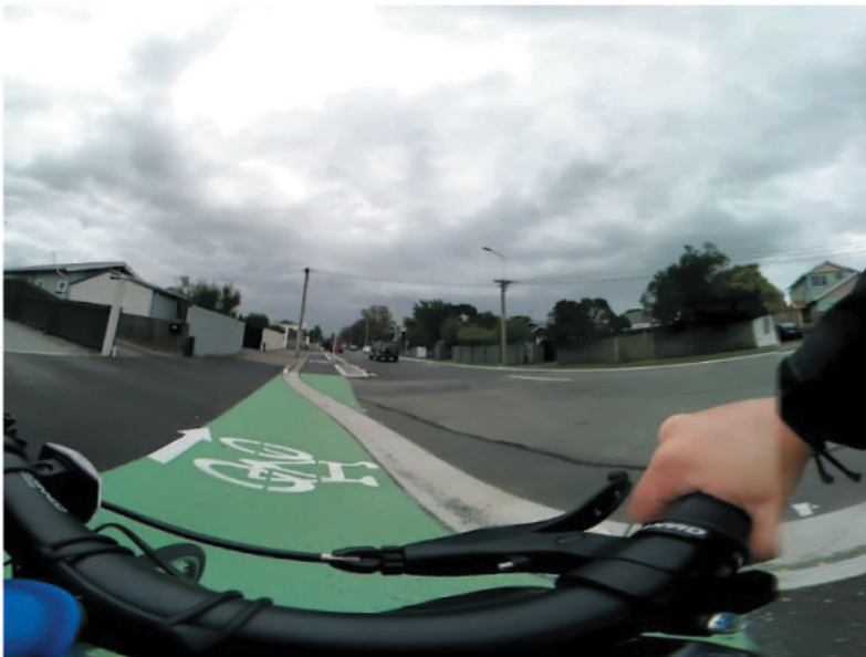
Figure 9. Bumpy design detail. Drainage kerb cuts through cycleway to connect disjointed street gutters. (Photo: The authors, 2018).
