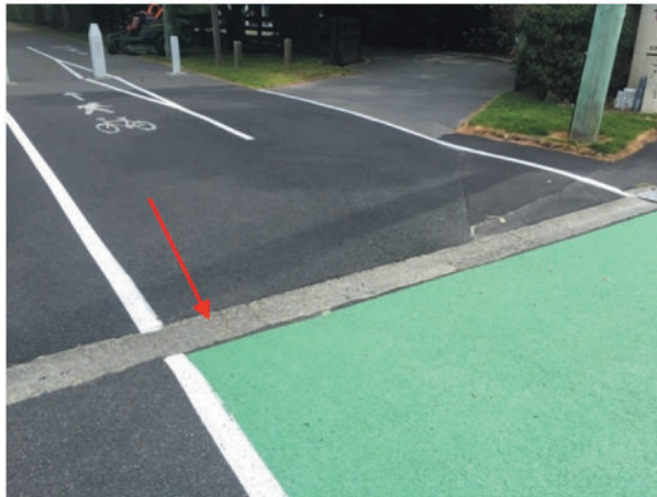
Figure 4a. Drainage kerb. (Photo: The authors, 2018).
