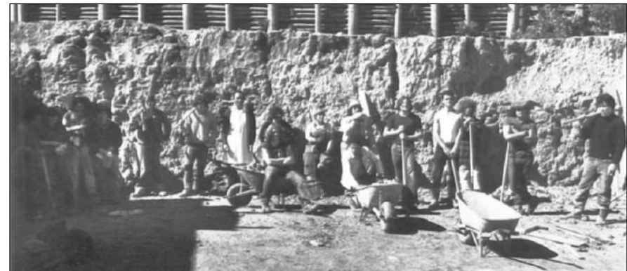
Figure 17. People constructing the foundations for Tapu Te Ranga.
