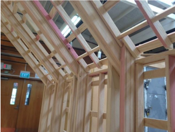
Figure 7. Mock-up #2 - wall/roof junction
