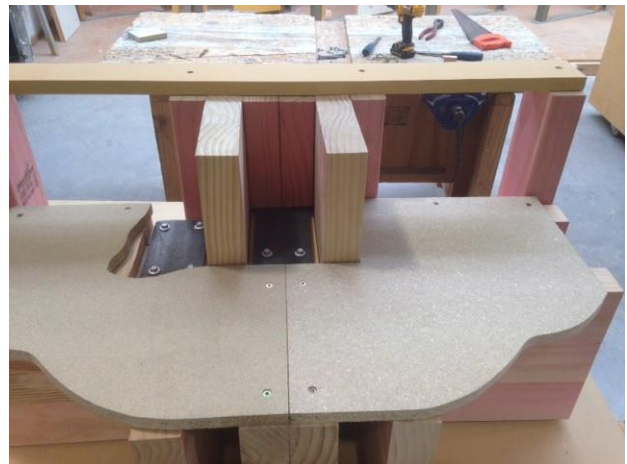
Figure 11. Mock-up #3 - floor cut-away, showing structural connectors
