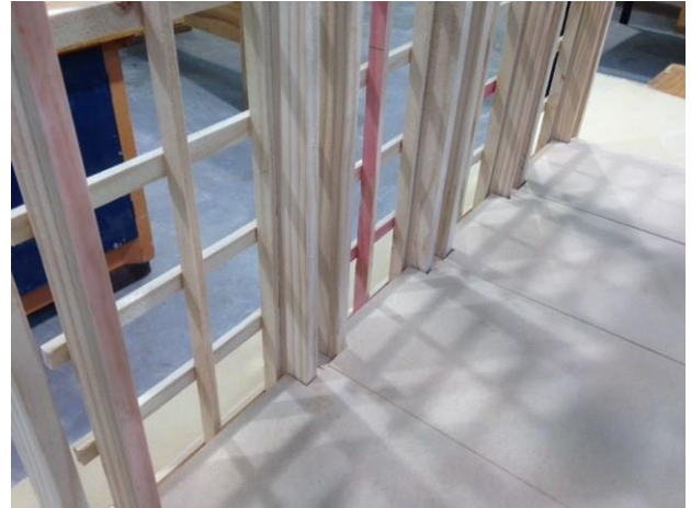
Figure 8. Mock-up #2 - Wall/floor junction
