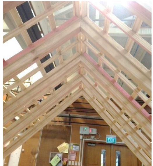
Figure 6. Mock-up #2 - underside of roof junction
