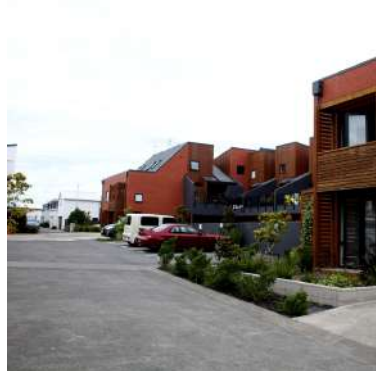
3 The communal spaces that could be used as children's play area are occupied by vehicles and parking spaces.
