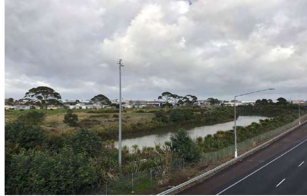
Main stormwater pond onsite
