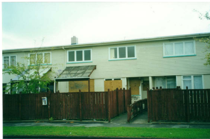
Figure 2. A photo showing a multi-story building in Aranui.
