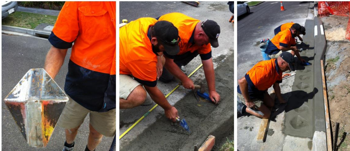
Figure 5-4 Sediment groove installation. Source: 2018 ZAM-WSUD Handbook.
