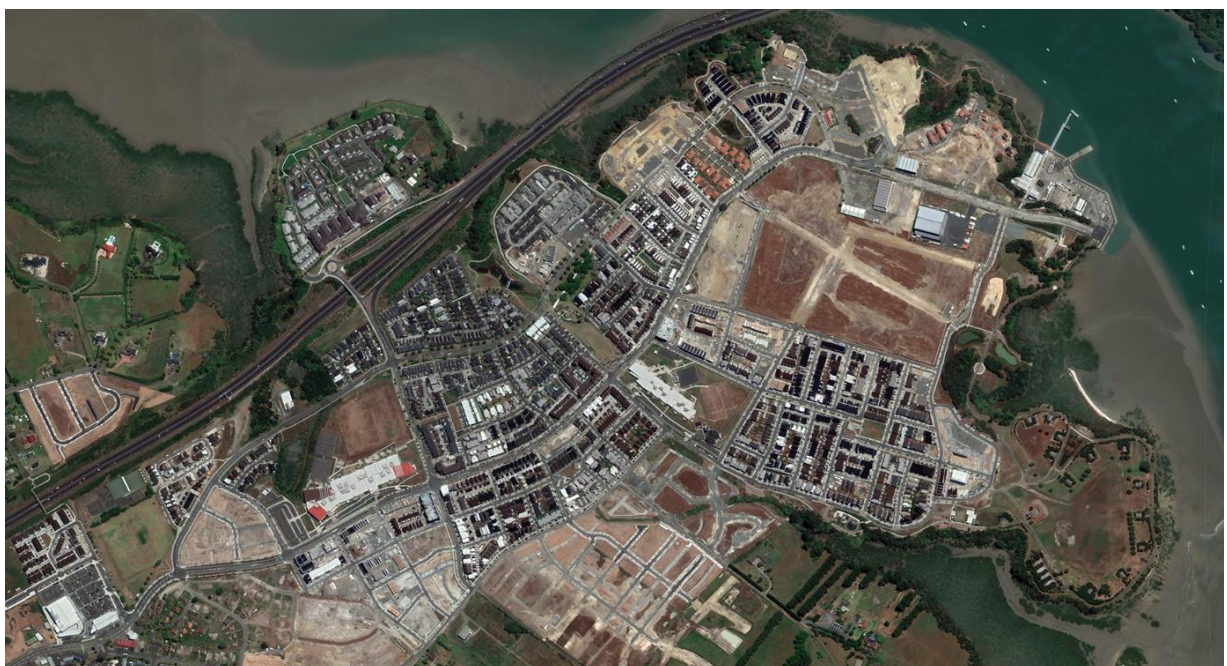
Figure 5. Aerial view of Hobsonville Point development as of end of 2018 (source: photomerge based on Google Earth images).
