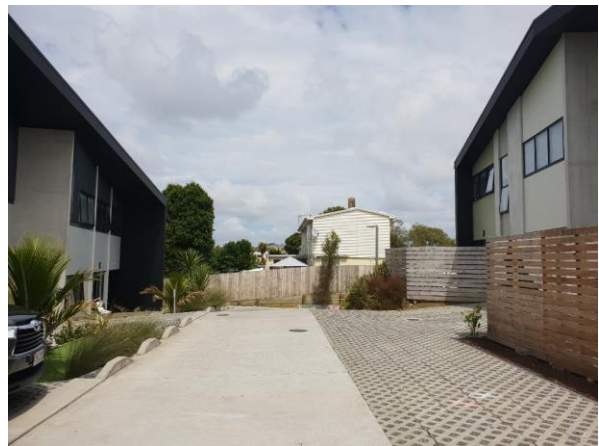
Figure 5: Shared internal laneway, including some permeable pavers to allow rainwater to soak through.
