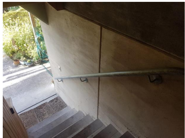
Figure 14: The ground floor walls of the homes in Earthsong are built with rammed earth, helping to reduce the embodied energy in constructing the homes.
