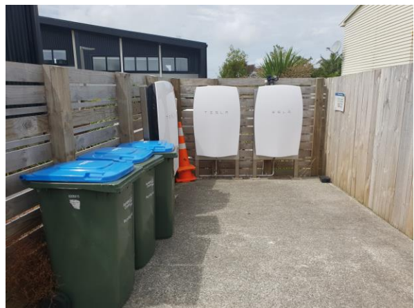
Figure 7: The development was the first to include Tesla power batteries, where energy produced from solar panels on the roof is stored and distributed to households.
