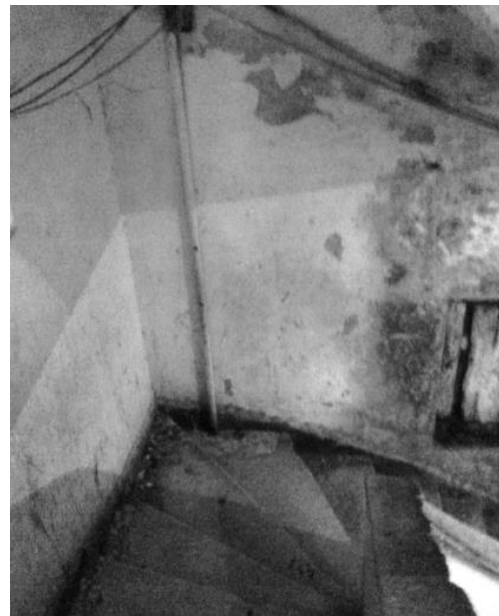
Figure 5.25: Prestes Maia building – inside of a communal stairwell for cleaning (photo credit: Caulkins, 2018, p. 83).
