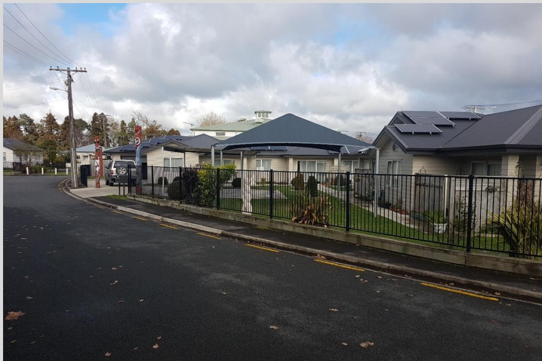
Figure 4.21: Kaumātua Village - buildings (stage two). The close-boarded timber fencing from stage one was largely replaced with more permeable fencing in this stage, allowing residents greater ability to see one another (e.g. if a neighbour has fallen). Stage two similarly has a shaded communal area, and solar panels visible on the roof. Also note the pou (carved posts) at the entrance to the site.
