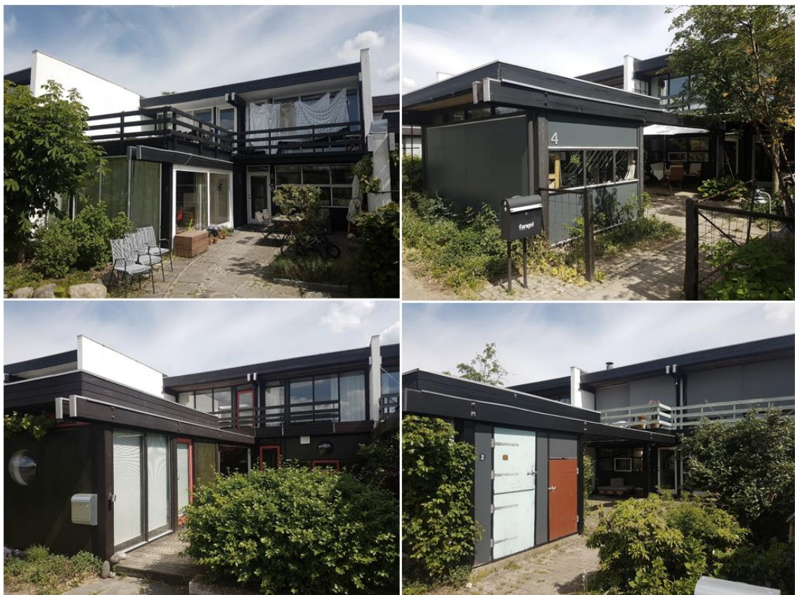
Figure 5.33: Sættedammen - four ground floor configurations. Residents have opted for different panels (i.e. walls, doors, windows or no panels) depending on their preferences, creating enclosed courtyards, additional rooms, or storage space (photo credit: author).
