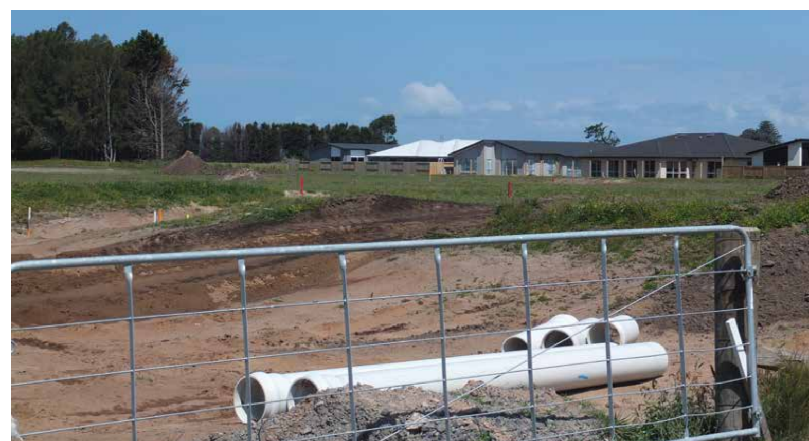
A greenfields SHA, showing earthworks and new homes.
